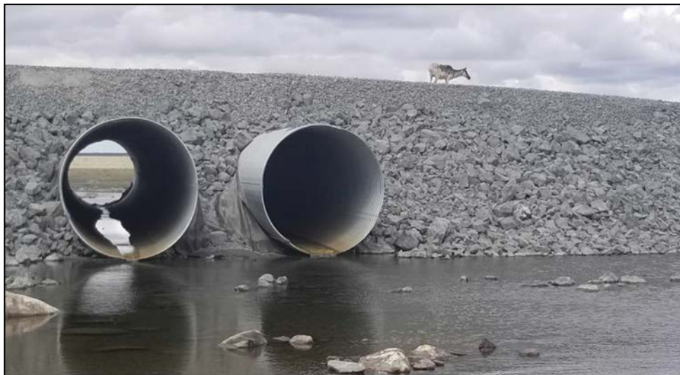
Photo 7-5: Adequate surface cover only present on the upper part of the slope. This substrate will need to cover the slope for approximately 100 m on either side of the road for each caribou crossing site.
