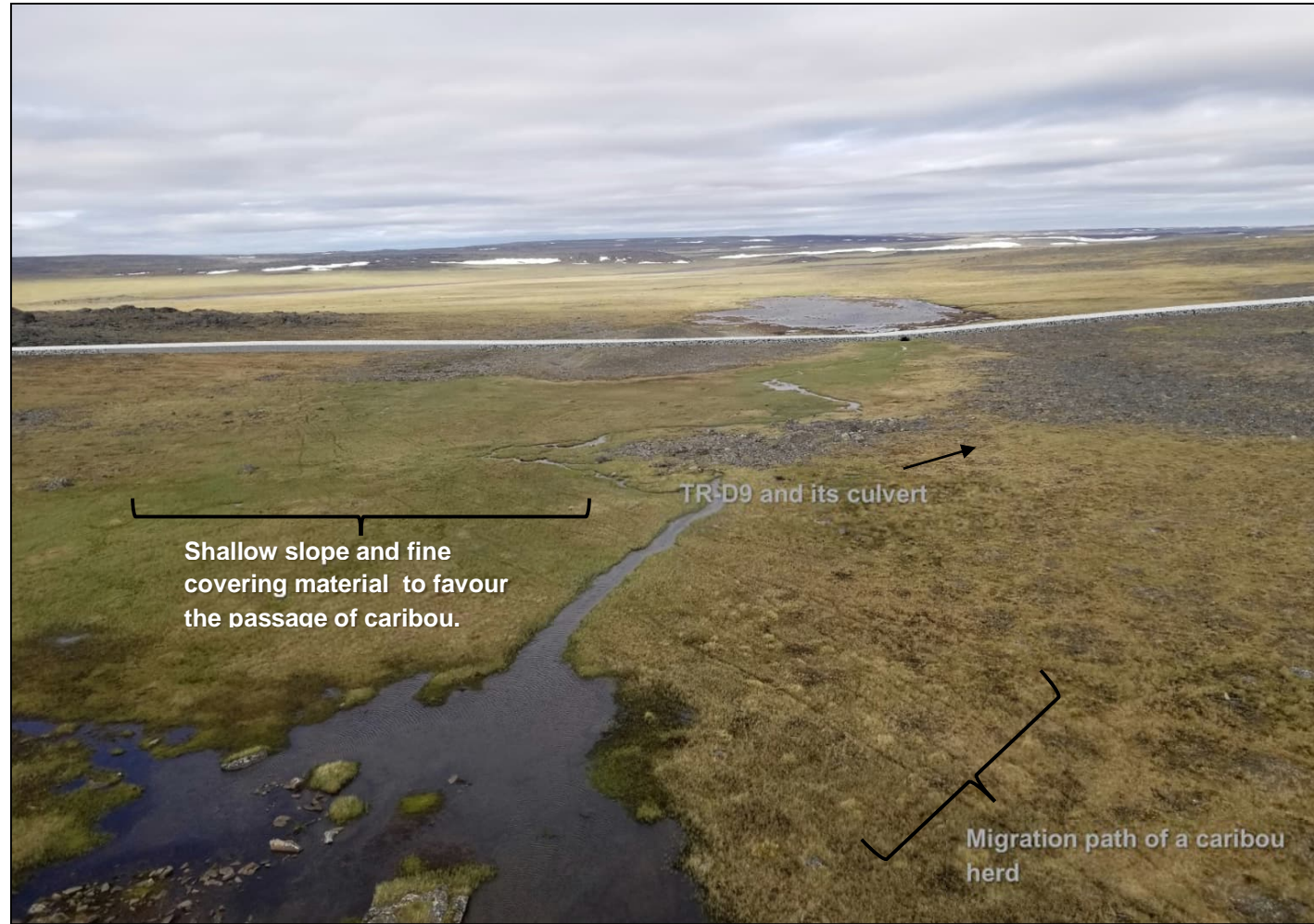
Figure 7-5: Visual simulation (profile view) of the Ivakkak-Delta road in the migration corridor of the caribou with the application of the mitigation measure to flatten the slopes
