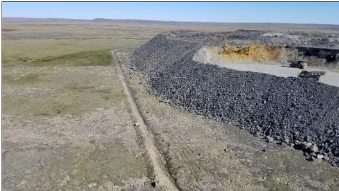
Photo 5-1: Examples of Non-Contact Water Diversion Ditch
