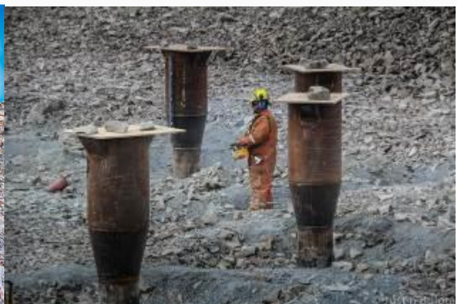
An example of a pile foundation
