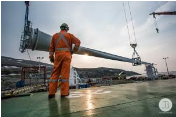
Unloading a 40 meter wind turbine blade from a ship in Nunavik.
