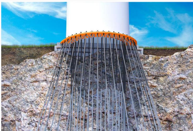
An example of a rock-anchored foundation
