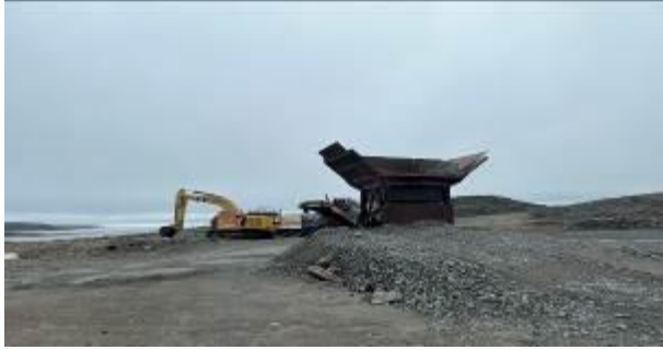
Crusher and equipment mobilized at the Quaqtaq quarry
