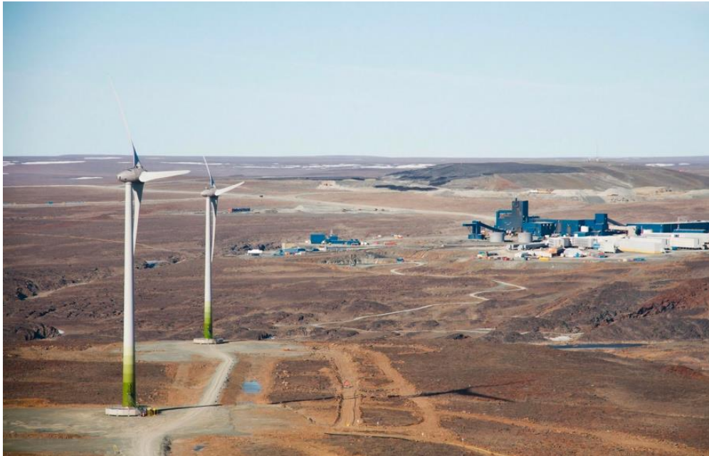
Figure 1-1: Photo of the two wind turbines installed on the Raglan Mine site
