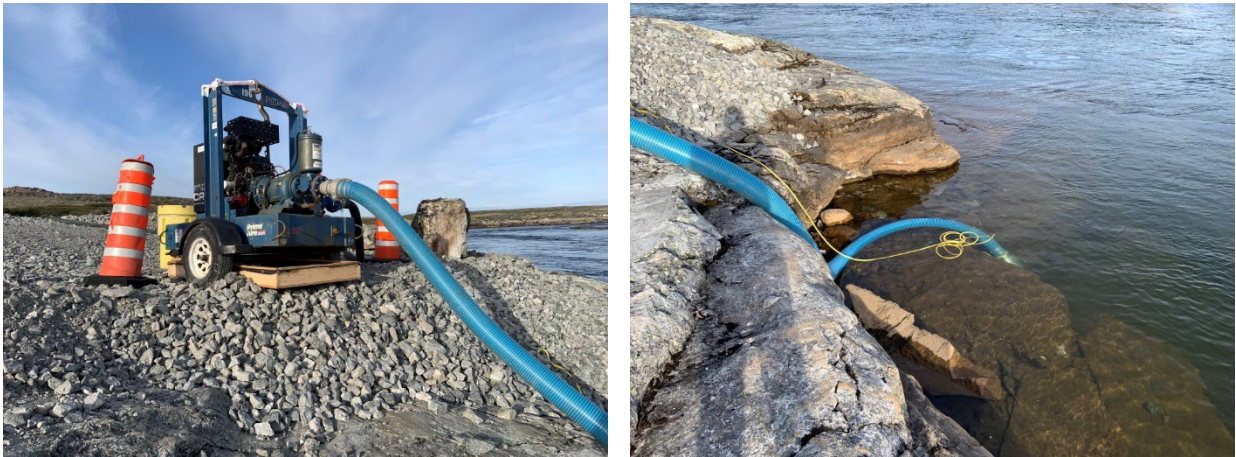
Figure 6 Installation of temporary water intake
