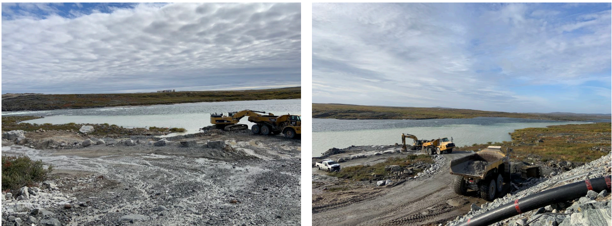
Figure 7 Formation of a plume following jetty excavation
