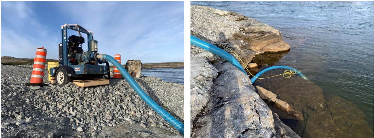
Figure 7 Installation of temporary water intake
